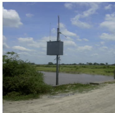
Level control in the Salado River, Santa Fe Province, Argentina.
